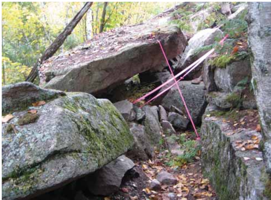
Trail damage caused by the 2006 earthquake.
