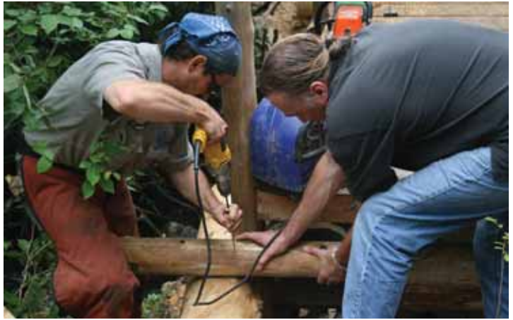
Volunteers secure portions of a bridge during construction.
